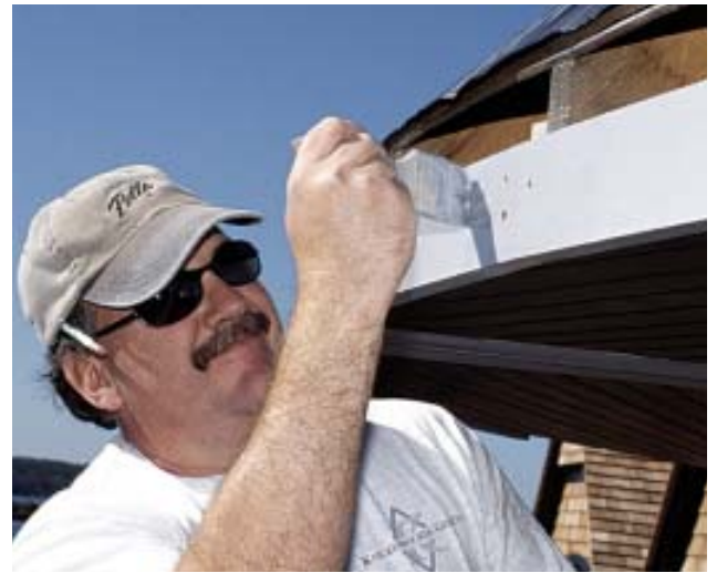
Figure 4. The trim was initially cut at the roof's pitch, then scribed for a closer fit with cedar shingles (top left). After installation (top right), the carpenters fine-tuned the joints with a random-orbit sander (left), then primed nail and screw holes to prevent weathering (above). The painter would later fill the holes with auto-body compound.
