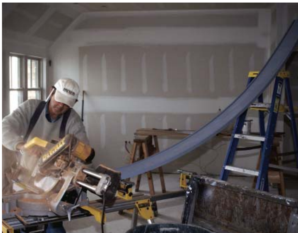
Figure 3. To produce the curved fascia, the crew first installed the T&G soffit (above), using a flexible straightedge held against the rafter tails to scribe the radius on the outer pieces. The soffit was then traced and the exact curve provided to the millwork shop. The curved fascia (above right), glued up from strips of Honduras mahogany, was made with a 1/2-inch-deep dado to accommodate any slight irregularities in the edge of the soffit. A stepladder allowed the cut man to reproduce the trim's installed position at the saw (right).
