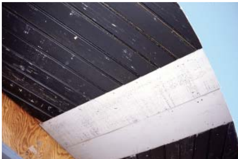
Figure 3. To produce the curved fascia, the crew first installed the T&G soffit (above), using a flexible straightedge held against the rafter tails to scribe the radius on the outer pieces. The soffit was then traced and the exact curve provided to the millwork shop. The curved fascia (above right), glued up from strips of Honduras mahogany, was made with a 1/2-inch-deep dado to accommodate any slight irregularities in the edge of the soffit. A stepladder allowed the cut man to reproduce the trim's installed position at the saw (right).
