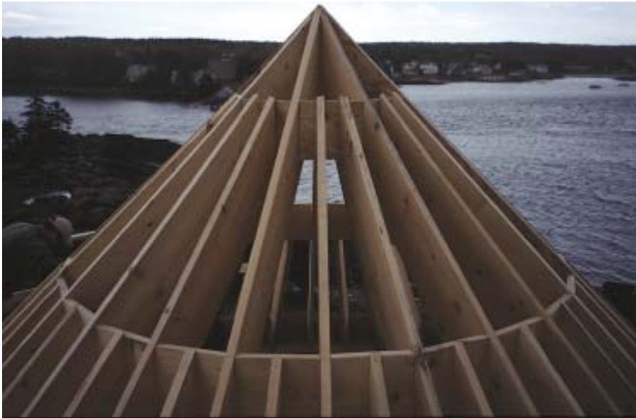
Figure 1. Accurate framing is critical for a good-looking curved trim job. In this case, the rafter tails lined up to within \frac{1}{8} inch, measured from the plate. The curved plates were built up from four layers of \frac{3}{4} -inch plywood, glued and screwed together.
