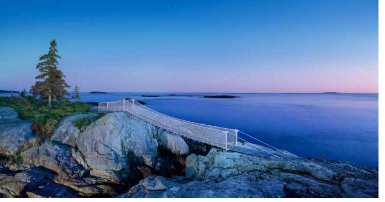
A bridge (above) of stainless-steel cables, galvanized posts, and cedar decking leads across a gap in the stone ledge where waves crash.
