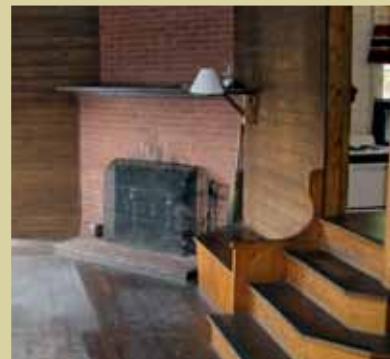
BEFORE – These “before” photos show how dramatically the cottage has been transformed. The third and fourth photos (counting down from the top) show the old kitchen.
