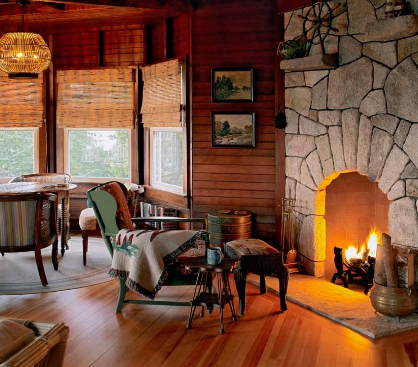
REMADE – The remodel’s biggest change was rebuilding the cottage’s brick fireplace (shown on p. 35) with local granite. Also shown here is a game table where the family builds puzzles and plays cards.
