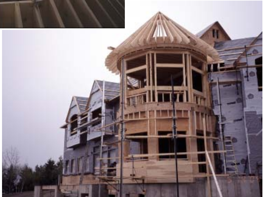
Figure 1. Accurate framing is critical for a good-looking curved trim job. In this case, the rafter tails lined up to within \frac{1}{8} inch, measured from the plate. The curved plates were built up from four layers of \frac{3}{4} -inch plywood, glued and screwed together.
