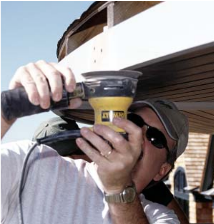
Figure 4. The trim was initially cut at the roof's pitch, then scribed for a closer fit with cedar shingles (top left). After installation (top right), the carpenters fine-tuned the joints with a random-orbit sander (left), then primed nail and screw holes to prevent weathering (above). The painter would later fill the holes with auto-body compound.
