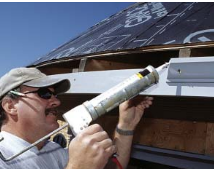
Figure 5. The crew positioned the crown molding so its top edge would be covered by the copper drip edge (top left). Quick-adjusting bar clamps kept the crown tight to the fascia while it was fastened (top right). To avoid gaps caused by seasonal movement, the carpenters used scarf joints. The cuts were spot-primed and the joints sealed with a healthy dose of caulking (above left), then fastened with stainless screws (above right).
